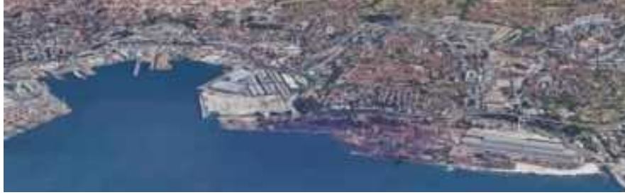
The PNRR interventions and "Pier VIII" of the Port of Trieste Trieste, 1 October 2025
